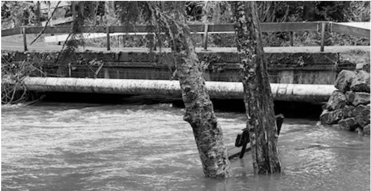
May creek bridge during the recent flood
