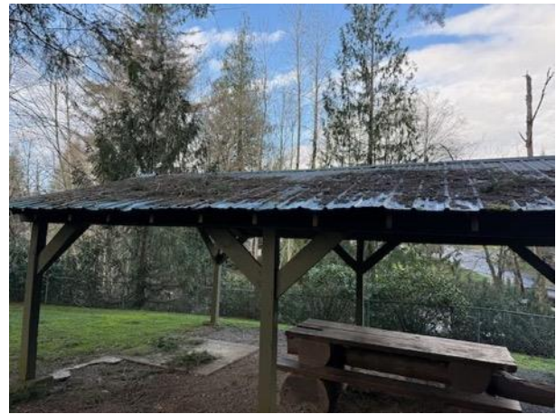
Roof should be kept clear of debris to avoid buildup and deterioration
