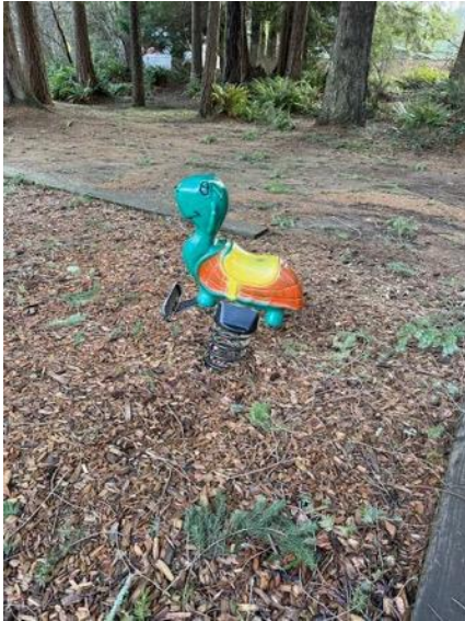
Rocker was loose and showing signs of rust and deterioration
